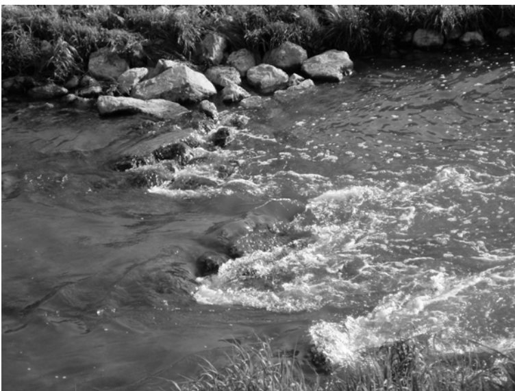
Figure 5. flat bed sill in detail
