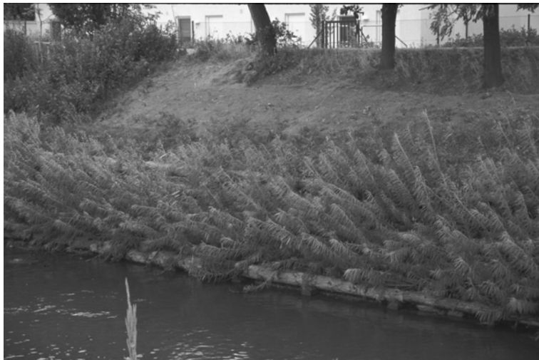
Figure 6. The vegetated crib-wall 5 month after construction.
