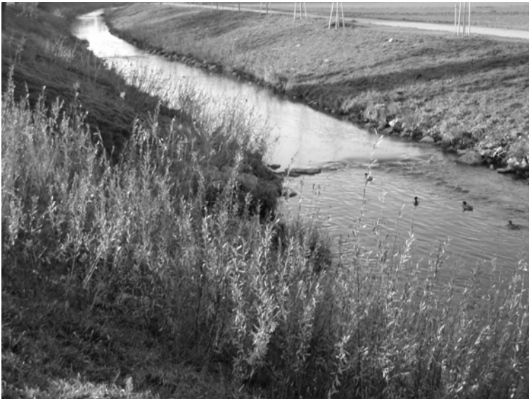
Figure 4. Series of new bed sills allow migration of fish and other river inhabitants again
