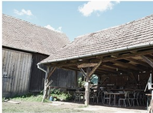
annex transformed into a pottery workshop
