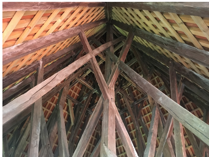
Timber Construction of the church tower
