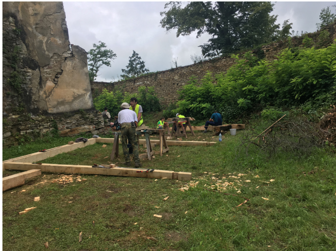
Creating timber joints
