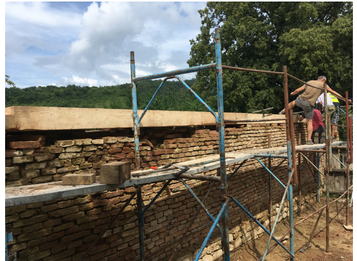
Placing the beam
