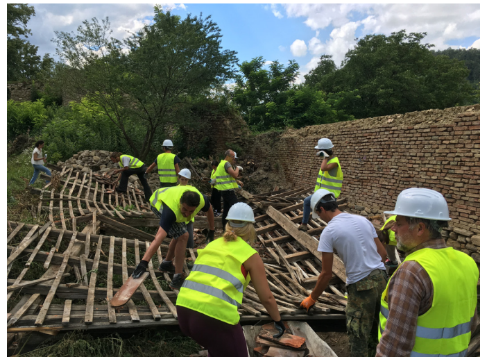
Cleaning the site
