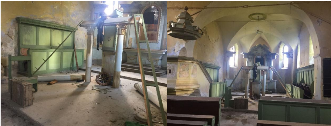
Figure 19 and 20, Photos inside from the Church in Pelisor.
