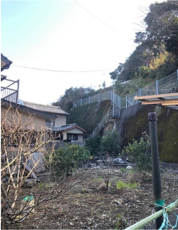
Picture 1 - Stairs, a part of the evacuation route (32°45'34.4"N 132°57'54.7"E)
