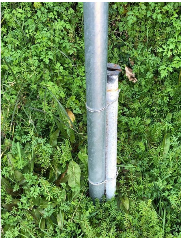
Picture 4 - Base of a portable light (32°45'31.8"N 132°57'56.2"E)
