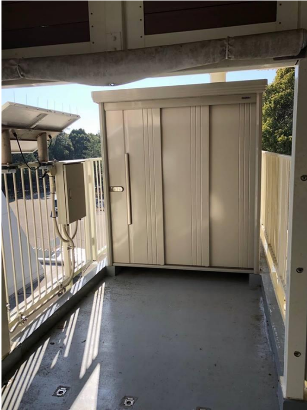
Picture 6 - A supplybox on top of a tsunami evacuation tower (33°01'20.4"N 133°00'46.9"E)
