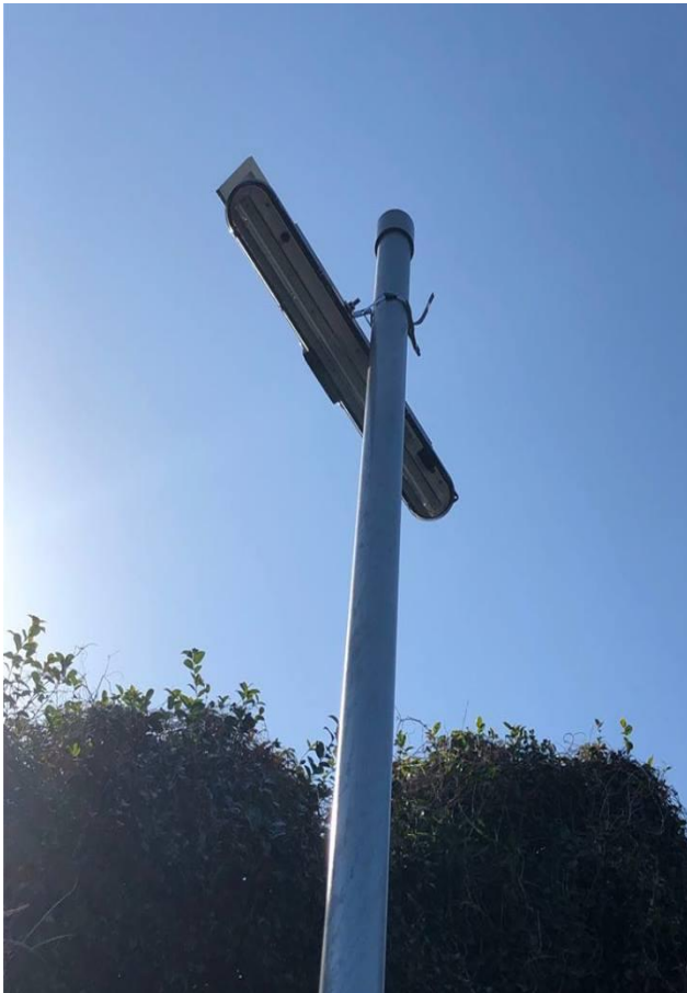
Picture 3 - A portable solar power light (32°45'31.8"N 132°57'56.2"E)
