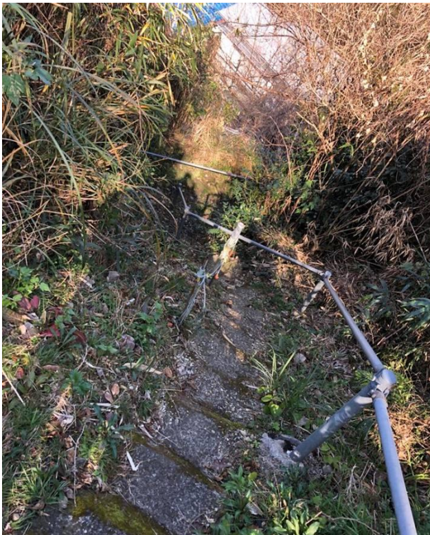
Picture 2 - Handrails and stoneplates to ensure the evacuation route (32°45'33.8"N 132°57'55.3"E)
