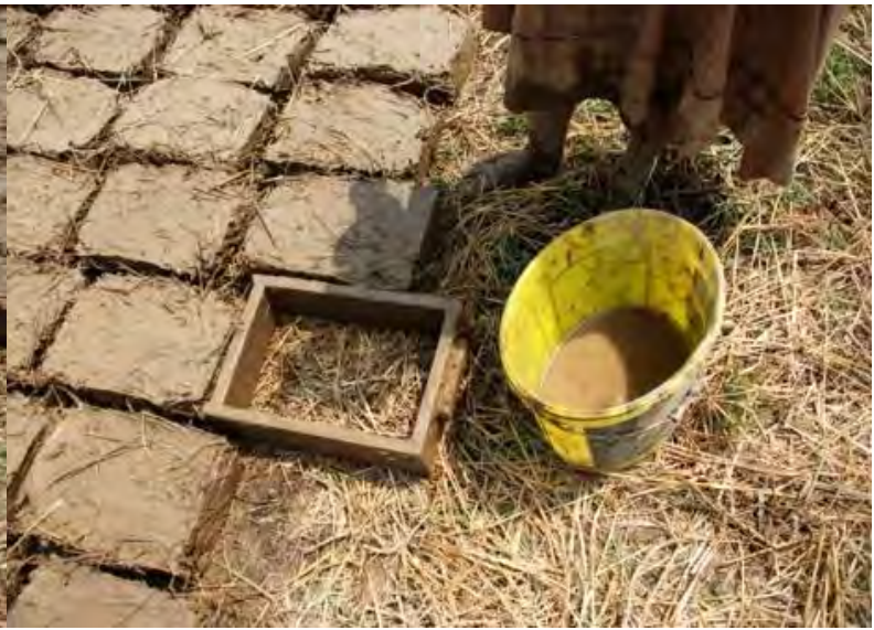
Preparing of chirpic bricks in Adamclisi village in Constanta county, Dobrogea
