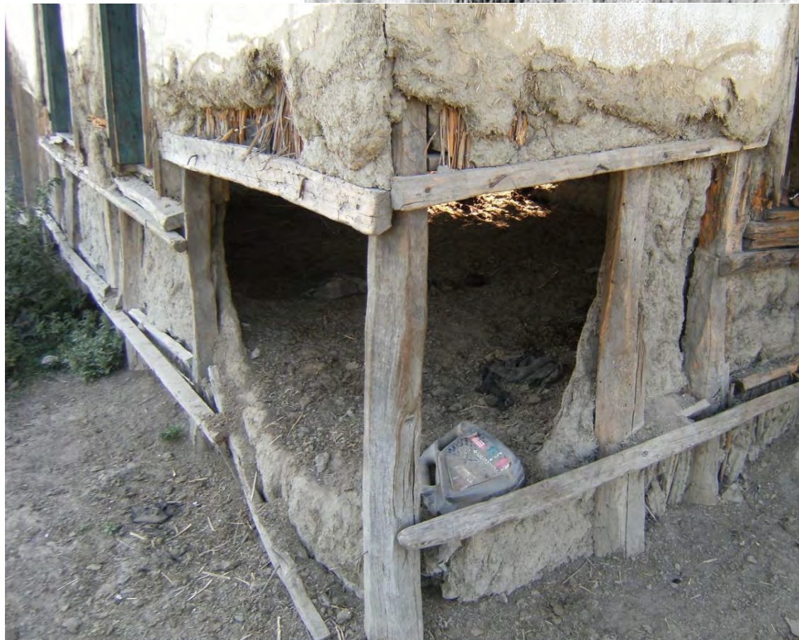
Rudimentary timber frames within a fork-type wall – Letea village
