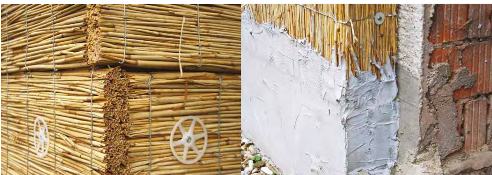
Pictures - External reed thermal insulation
